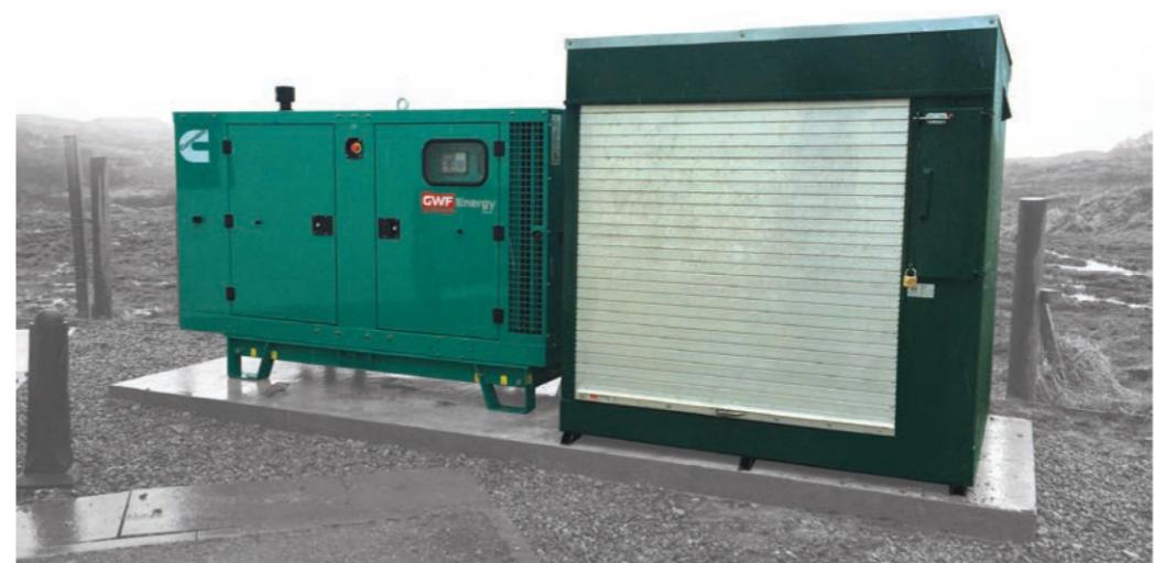
In a remote and unmanned location sourcing fuel was critical. The addition of a fully bunded fuel store offered the ability to source fuel in smaller quantities in case of emergencies. This was one of three set-ups installed on the Scottish Isles of Luing, Lismore and Gigha.
